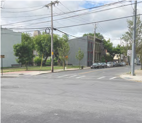
existing conditions: Lark Street / Clinton Avenue intersection
