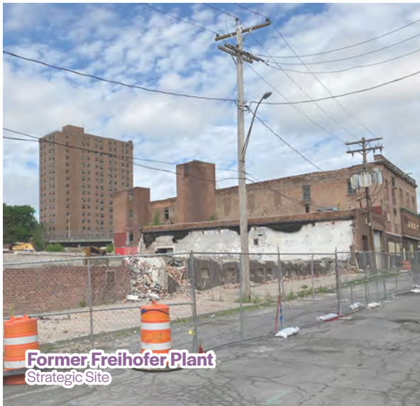
existing site conditions as of May 2020
