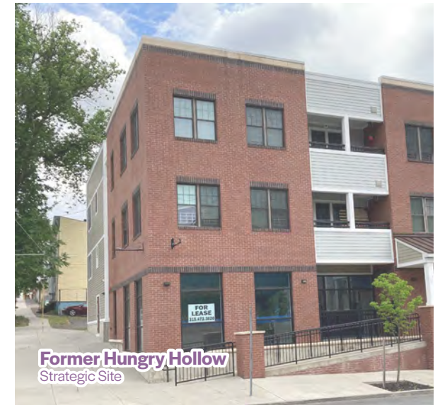
existing former Hungry Hollow building
