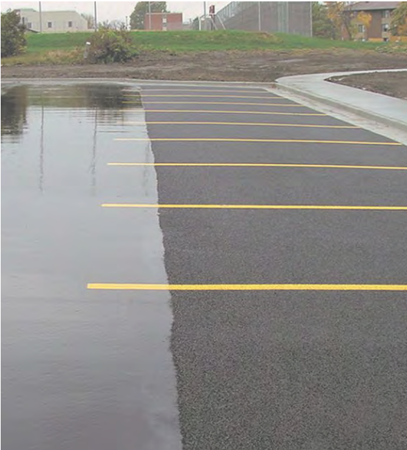
example of porous pavement
